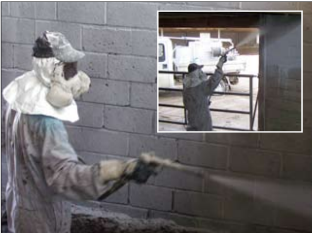
Figure 5: Example of whitewashing of a stable with milk of lime. Milk of lime may also be applied by brush or other suitable technique (Belgium).
