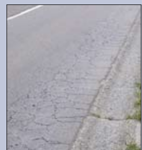
Oxidation cracking
